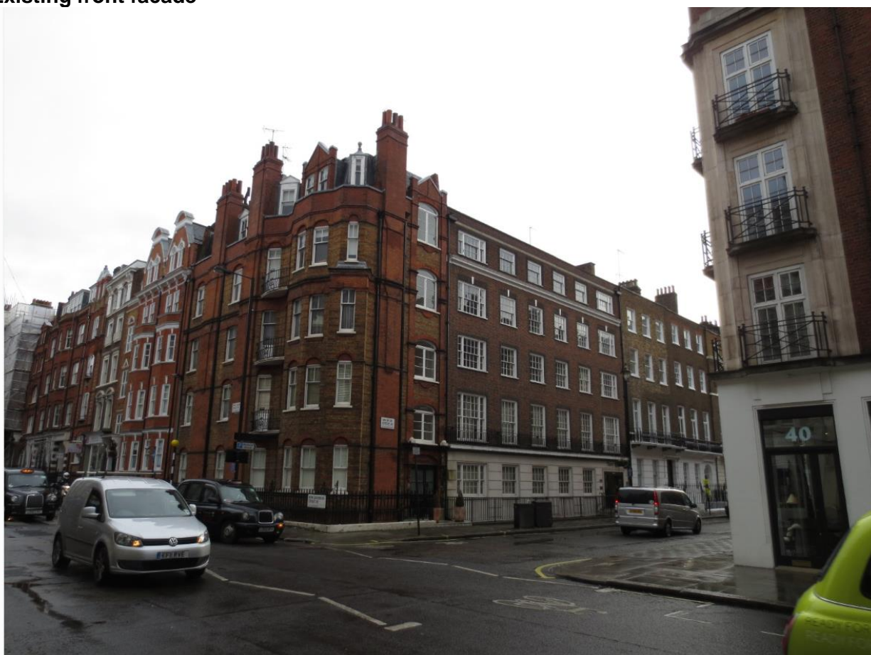
Existing front facade
